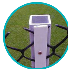
Securing the mesh to the post using a counter slat
