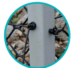
Installation of tension wires on posts
